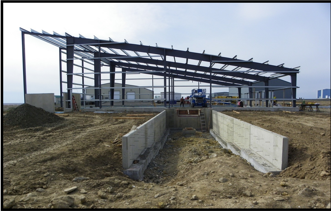
A new meat processing facility under construction.
