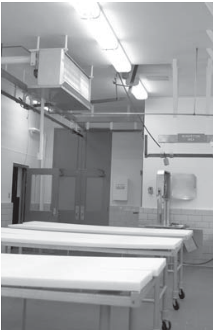
Figure 5. Overhead refrigeration and/or condensation units may be a source of L. monocytogenes or Listeria spp. if they drip onto ready-to-eat processing areas.
