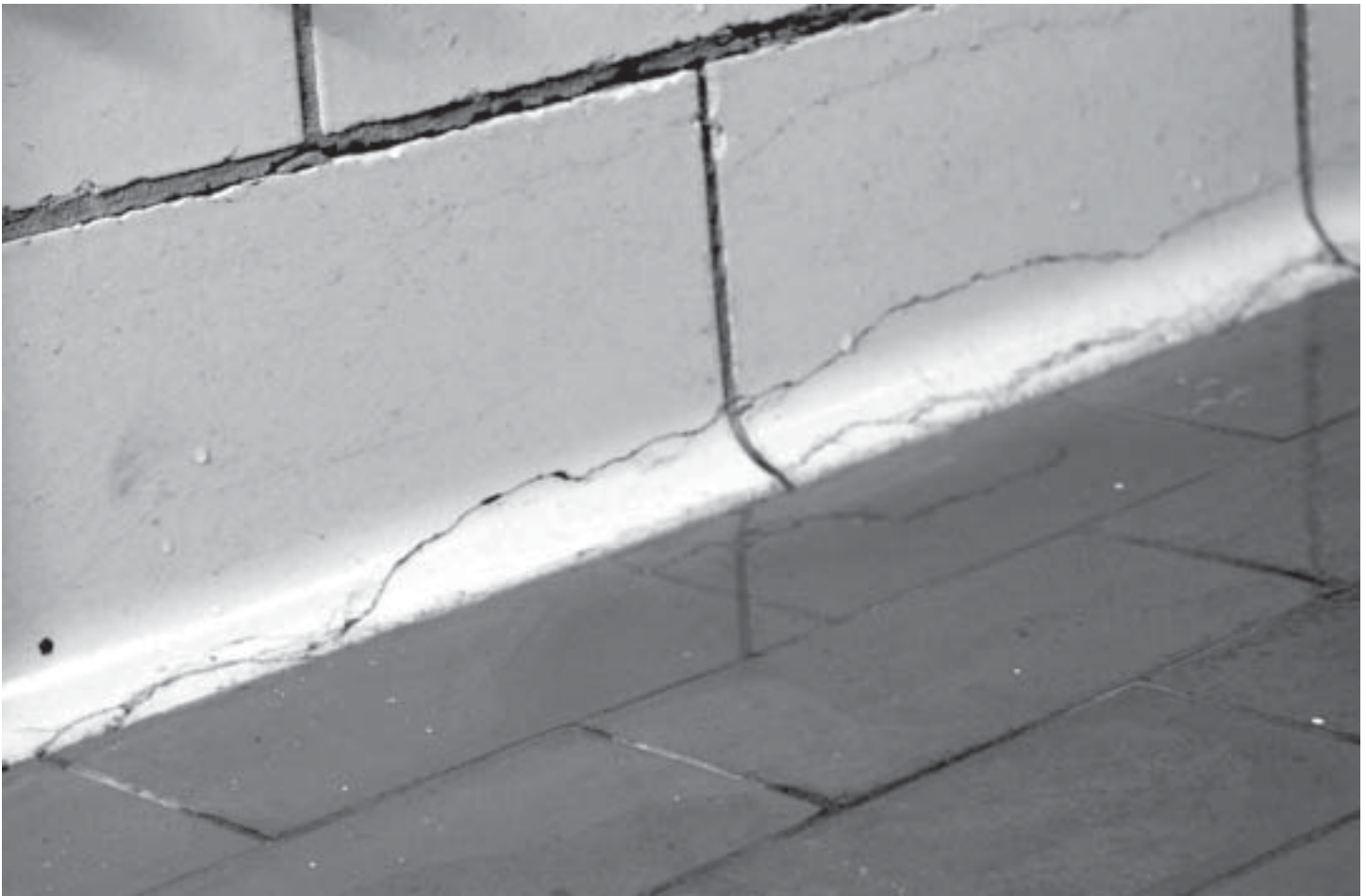
Figure 20. Cracks in flooring material may be a potential site of L. monocytogenes contamination.
