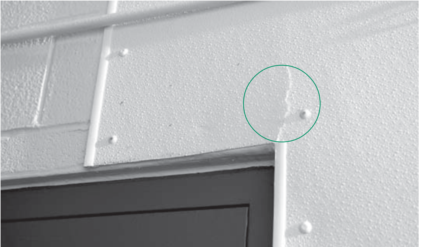
Figure 17. Cracks in wall boards may allow bacteria and moisture to become trapped in the insulation, creating an environment that allows for growth of L. monocytogenes .
