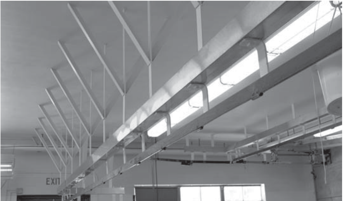
Figure 18. Since L. monocytogenes can survive in dry environments, pay careful attention to or replace difficult-to-clean overhead structures and light fixtures.
