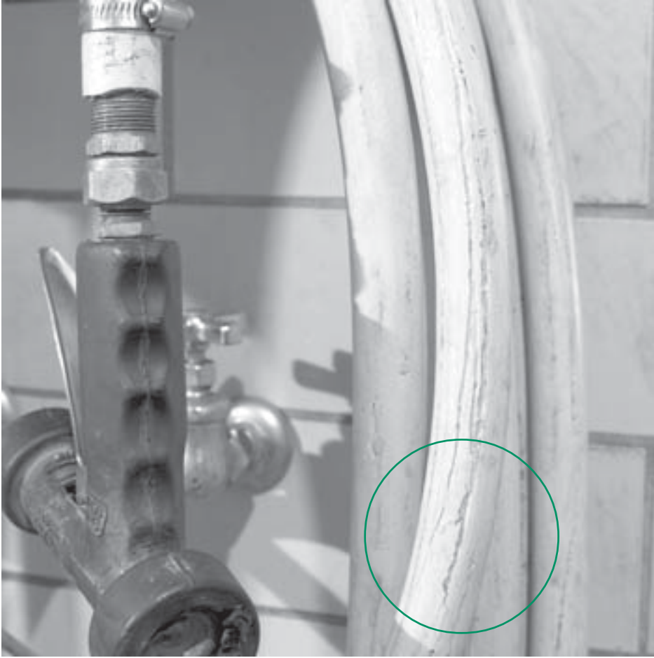
Figure 11. Since they come in direct contact with floors and drains, cracked hoses may be a source of L. monocytogenes contamination in processing establishments.
